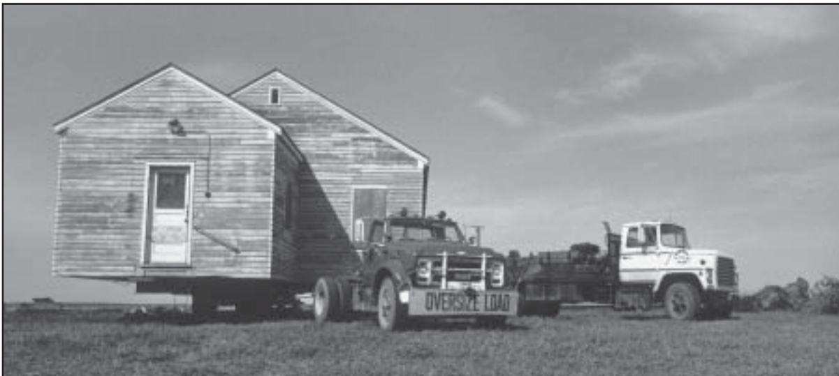
The Cornwell farm house loaded on a rig of steel beams and wheels for its move from the farm to the town of Rolfe in 1989. Northeast corner, Section 14, Roosevelt Township.
