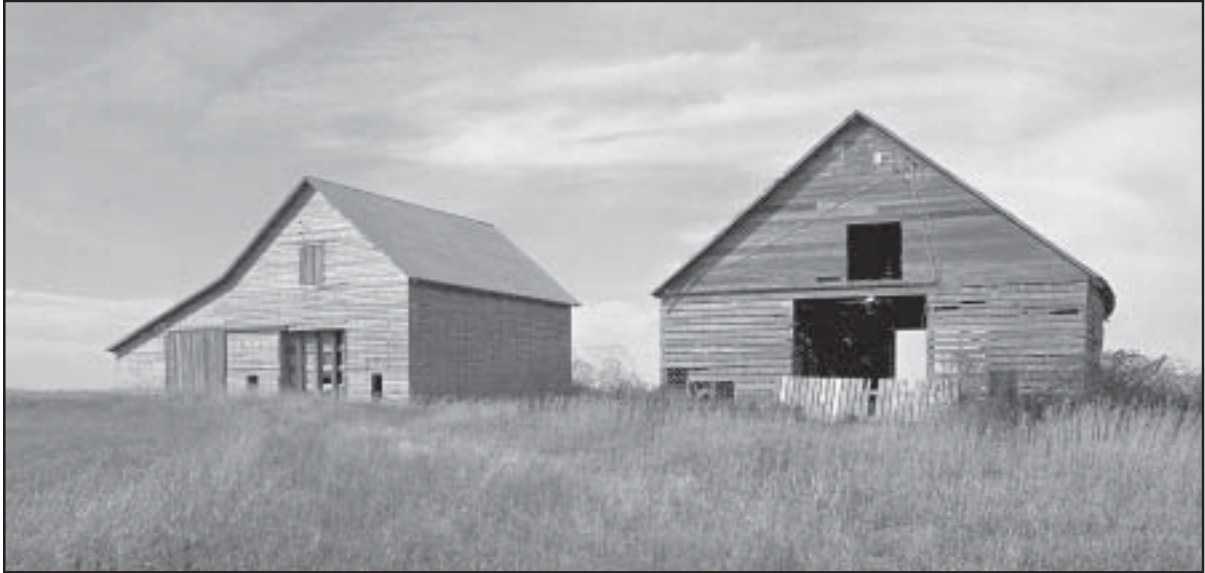
The last buildings at the farm where the Jordan family lived on the south side of Section 10, Roosevelt Township, 1994. Both buildings have been razed, and the land is used to grow corn and soybeans.
